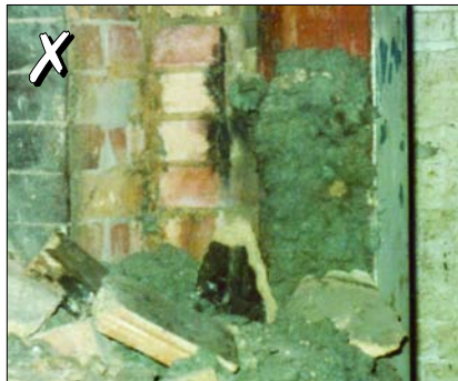
Limpet/sprayed asbestos
