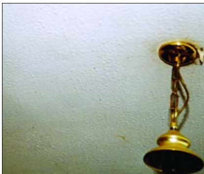
Textured coating on a ceiling
