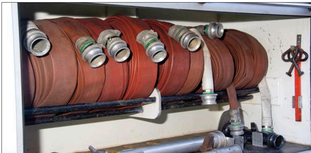
**Figure 39** Firefighting hoses conspicuous locations along the escape routes, such that nobody in the storage area needs to travel more than 30 metres to reach one. Unless the location of an extinguisher is self-evident, its position needs to be identified by appropriate safety signs. Such signs should comply with the Health and Safety (Safety Signs and Signals) Regulations 1996 or BS 5499-1.<sup>53</sup>
