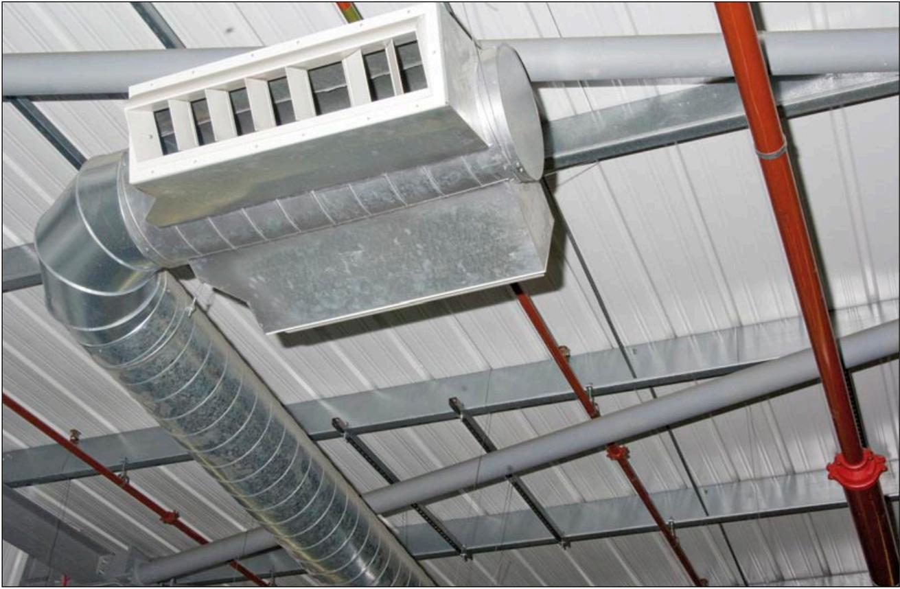
**Figure 22** Hot air heating system
