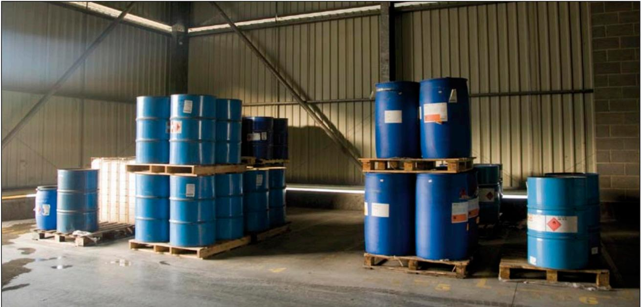
**Figure 28** A purpose-built, bunded chemical drum store
