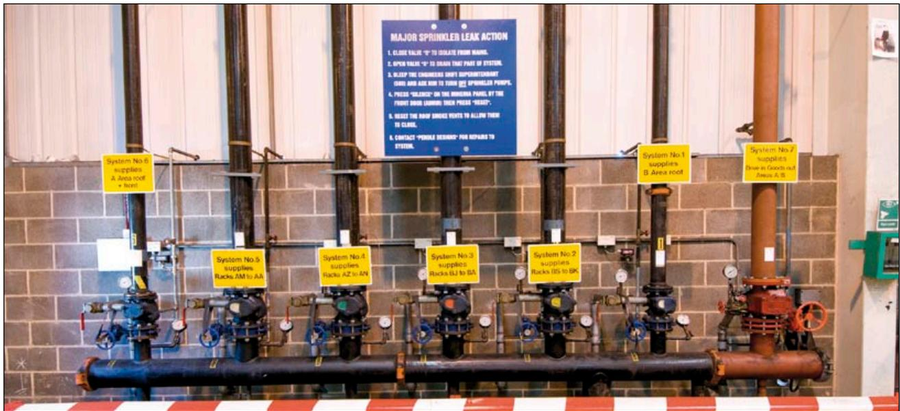
**Figure 41** Manifold for a sprinkler system
