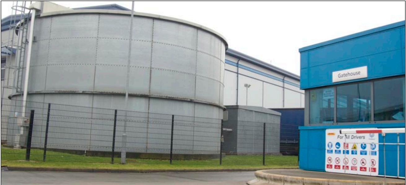
**Figure 42** A firewater tank
